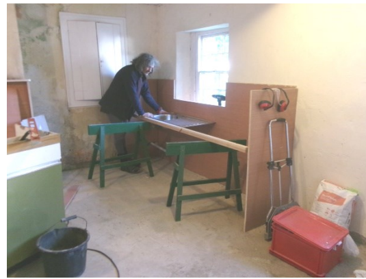
Rowan working on the kitchenette.
