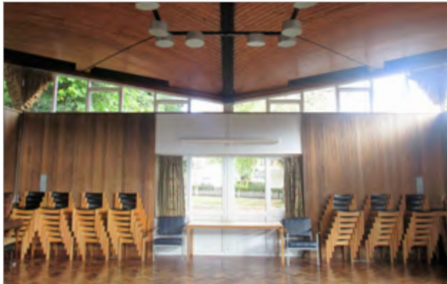
Clerestory windows below the hyperbolic paraboloid roof
