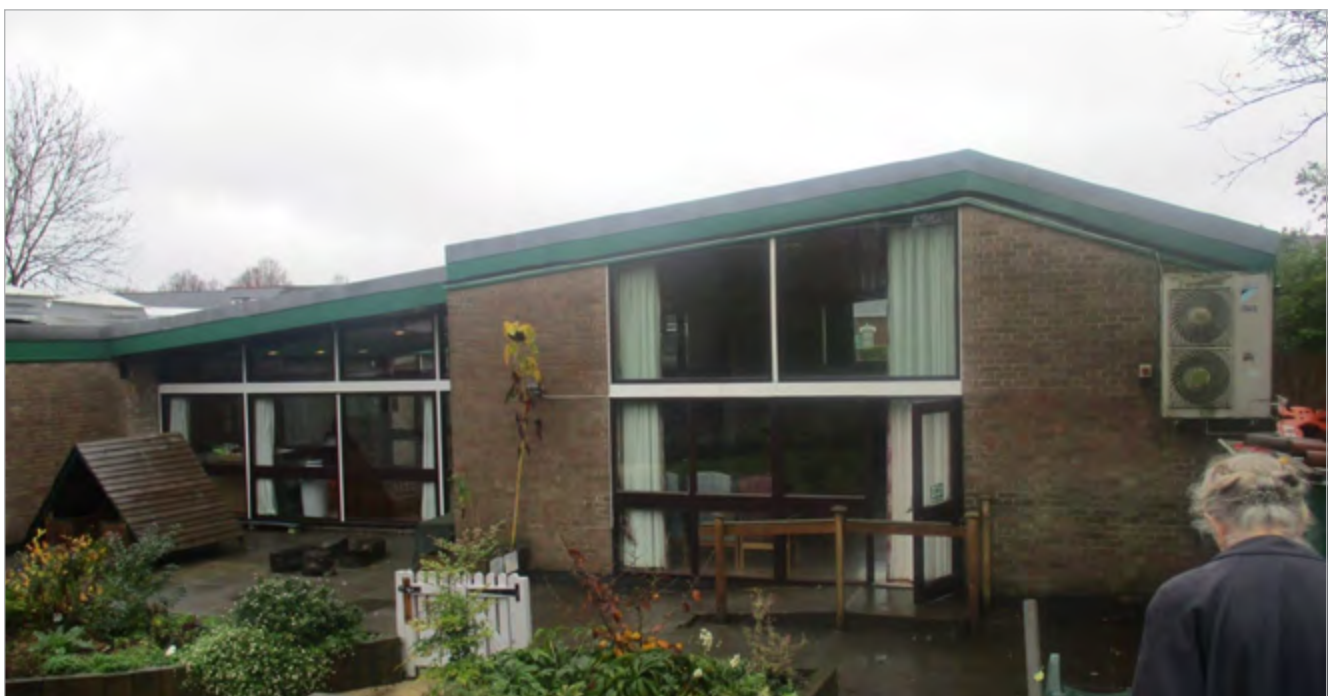
Rear view showing insect friendly garden, the 'glass walls' admired by Pevsner, now all double glazed, and (top right) external air source heat pump unit
